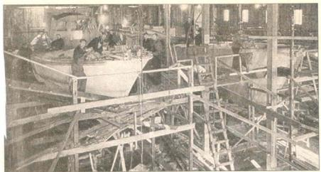
In these photos, two subchasers are under construction inside the buildings of the Perkins & Vaughn shipyard. Can anyone identify these workers?
