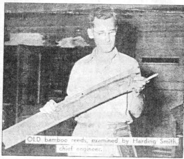
Harding Smith checks the reeds, which are used to keep the yarn separate as it feeds onto the loom.
